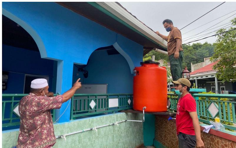
**Gambar 4. Pemasangan Tandon *Rainwater harvesting***
